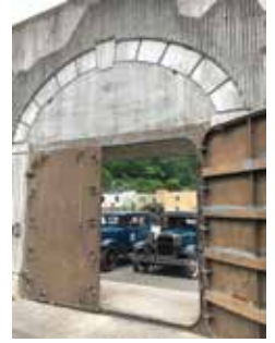
Floodwall in Matewan, W.Va.
